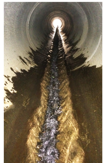
Mussel-rope in Culvert
