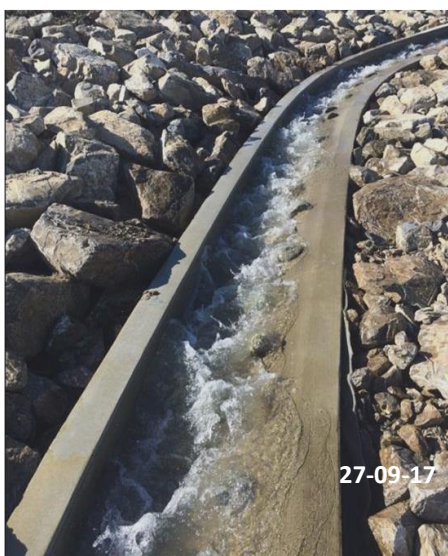
1 Failed Fish Pass
