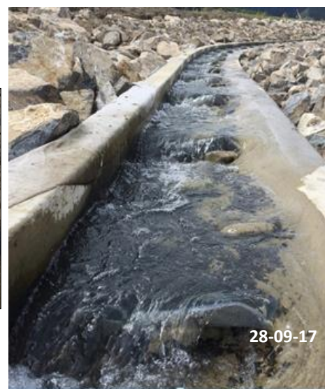
2 Remediated Fish Pass
