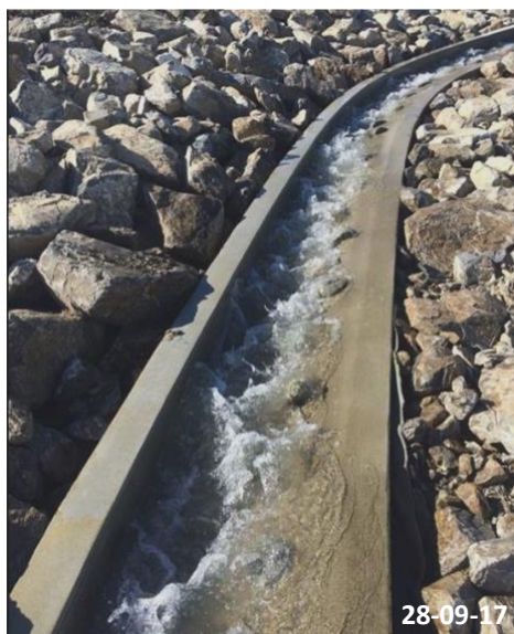
Figure 2. Failed fish pass
