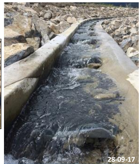
Figure 1. Retrofitted Fish Pass
